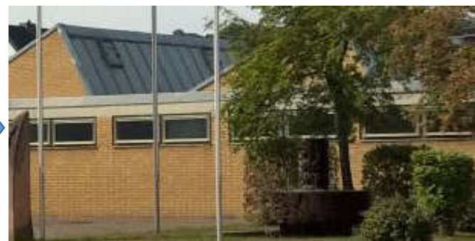
The building with workshops – named „Building M“
